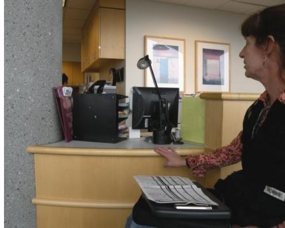
Figure 17: Computers and miscellaneous items block access to lower reception desk.
